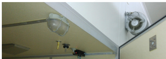
Figure 1 A hole drilled in the door and protected with a metal plate allows the insertion of the calibration probe close to the temperature sensor.
