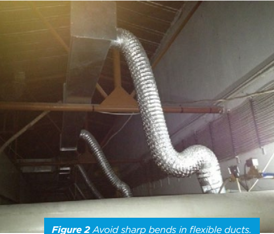
Figure 2 Avoid sharp bends in flexible ducts.
