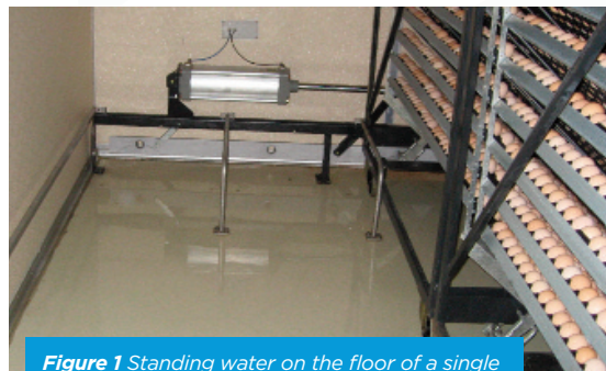
Figure 1 Standing water on the floor of a single stage setter at the end of the sealed period.
