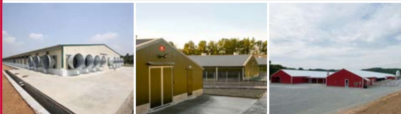
Figure 2.4 Houses with a low biosecurity risk showing concrete areas and no vegetation around the immediate perimeter of the house.
