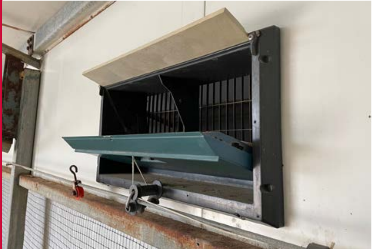
Figure 6.10 Example of a good-quality air inlet.
