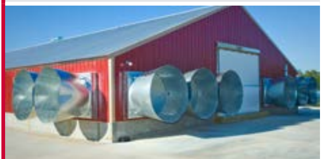
Figure 6.17 Example of a typical tunnel-ventilated house.
