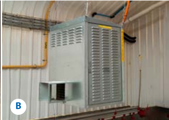
Figure 6.3 Examples of different house heating systems: canopy brooder (A), box heater (B), space heater (C) and hot water air heater (D).
