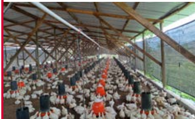
Figure 6.4 Example of an open-sided house.
